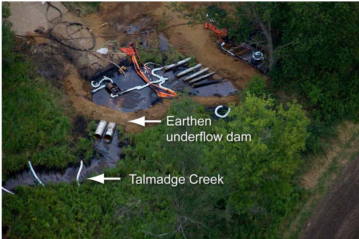
Figure 10. Underflow dam on Talmadge Creek on July 30, 2010.
