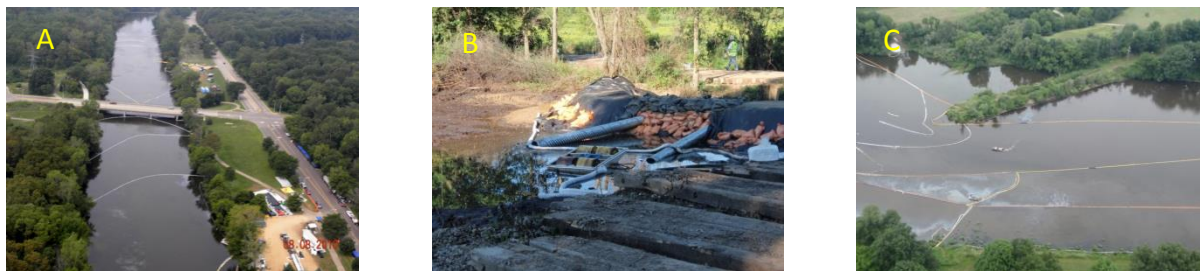
Figure 3. Oil collected over time with different methods: A, conventional floating absorbent boom; B, inverted weir dam in Talmadge Creek; and C, new agitation toolbox technique (photos by Weston/START).
